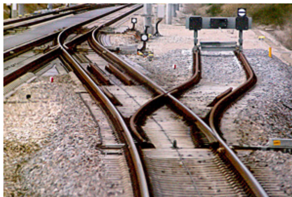
Railway points photograph by S. Terfloth
